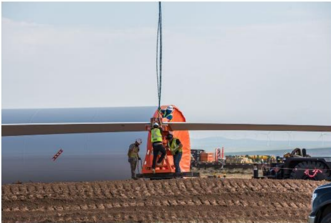
Construction workers unload a turbine blade at a wind farm in Encino, New Mexico. Photographer: Cate Dingley/Bloomberg
